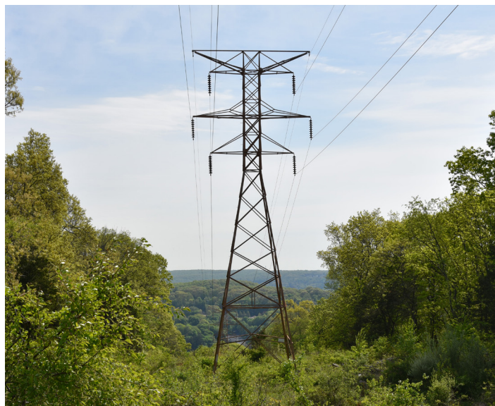
Typical existing lattice steel structure in Derby
