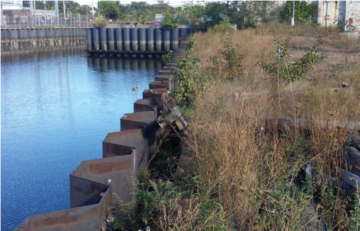
Photo 1 Phase 1 Bulkhead, minor coating deterioration inshore face
