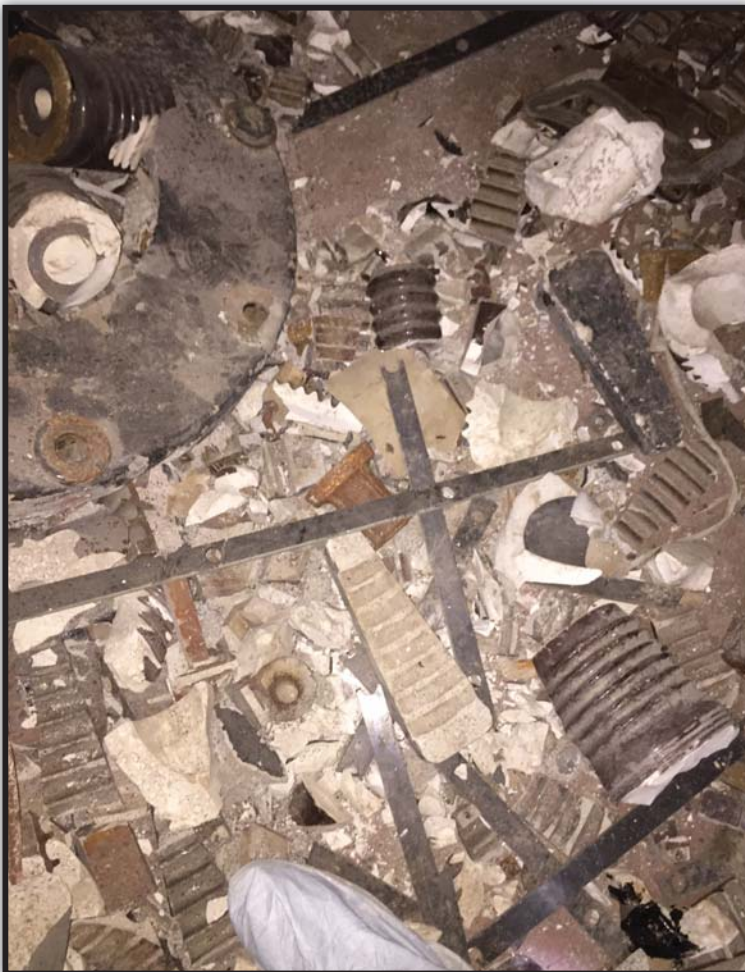
PHOTO 10. English Station - Second Floor, Switch Cell Area.
