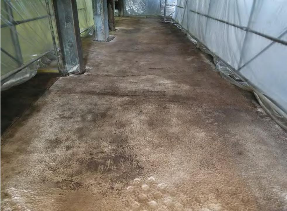
Photo 25: Typical poly-sheeting protection inside containment covering scaffolding (West Area) following scabbling and surface vacuuming and wash.
