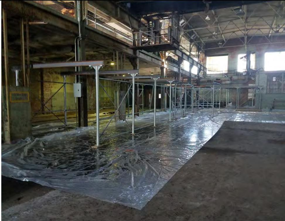
Photo 21: Scaffolding being erected on poly-sheeting .
