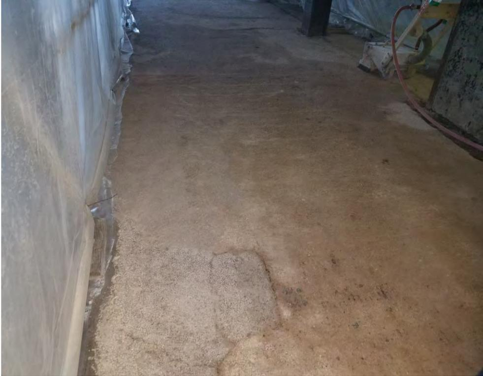
Photo 23: Typical poly-sheeting protection inside containment covering scaffolding (West Area) following scabbling.
