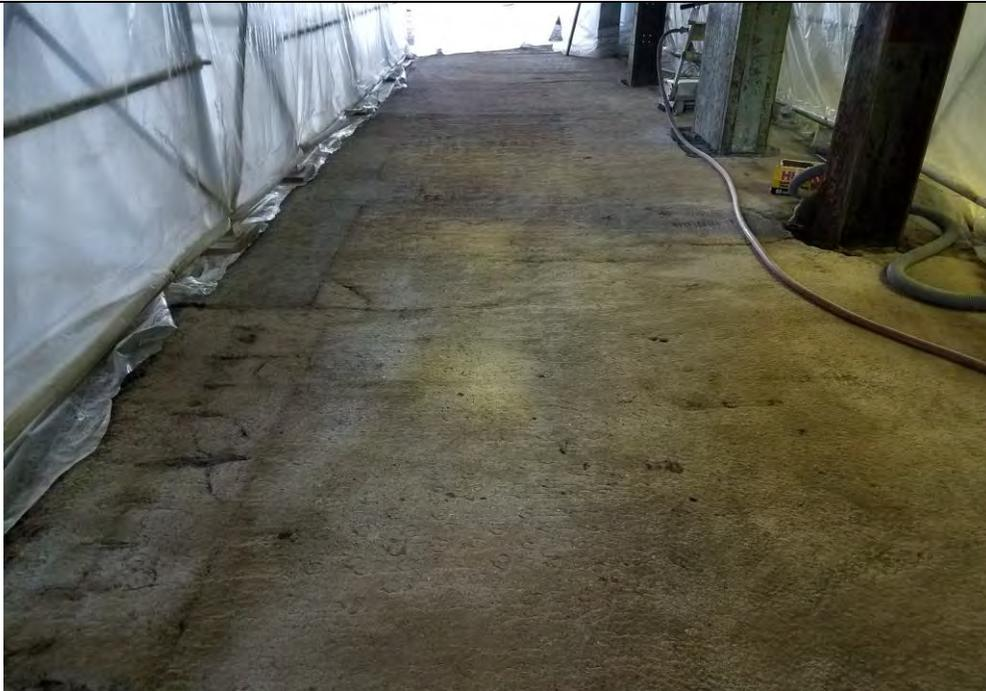
Photo 24: Typical poly-sheeting protection inside containment covering scaffolding (West Area) following scabbling.
