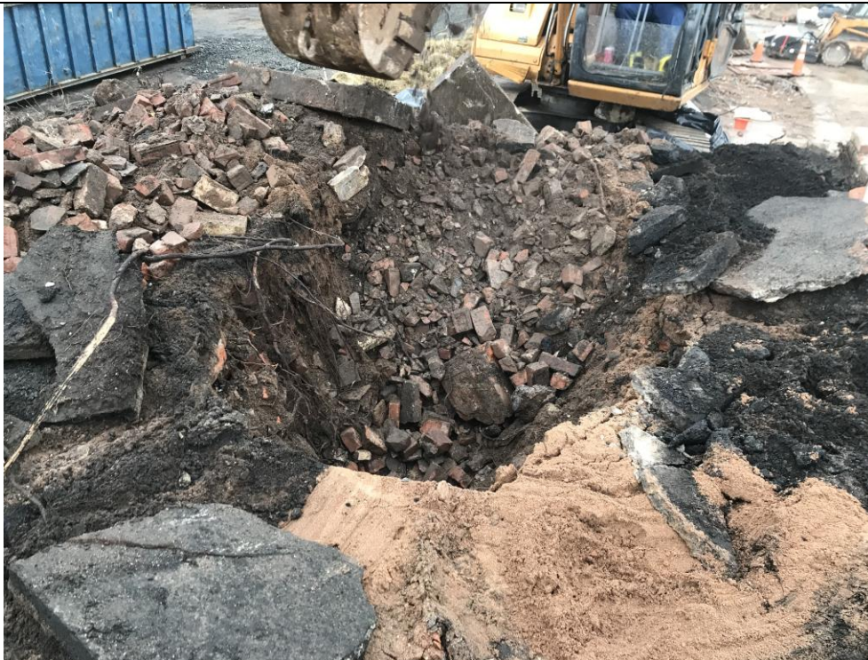
Photo 4: Test pit excavation and sampling at 5-foot depth.
