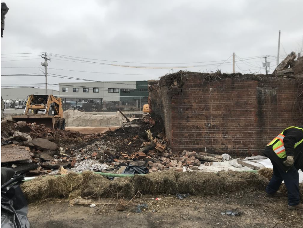
Photo 6: South side of filled platform wall prior to material load out.
