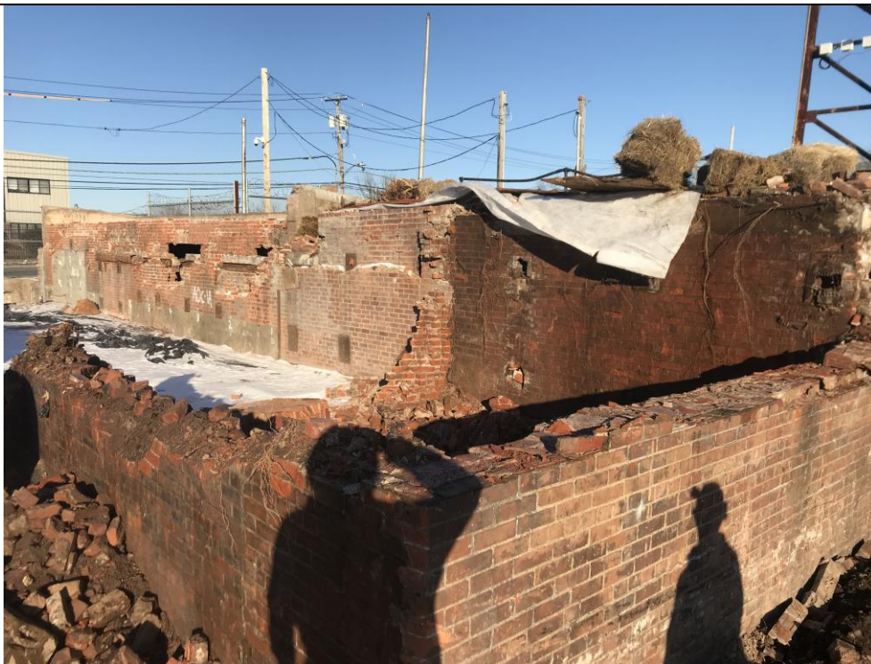
Photo 8: Filled platform area after material loadout and prior to brick support wall demolition.
