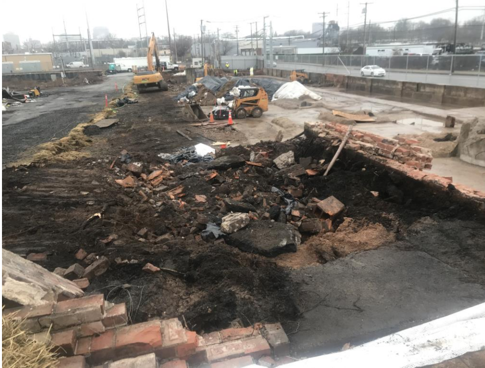
Photo 7: Top view of filled platform prior to material load out.
