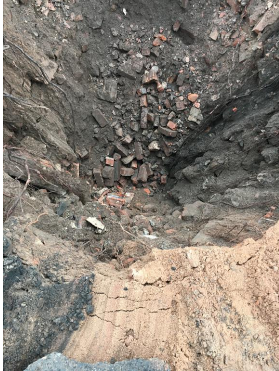
Photo 5: Test pit excavation and sampling at 9-foot depth.
