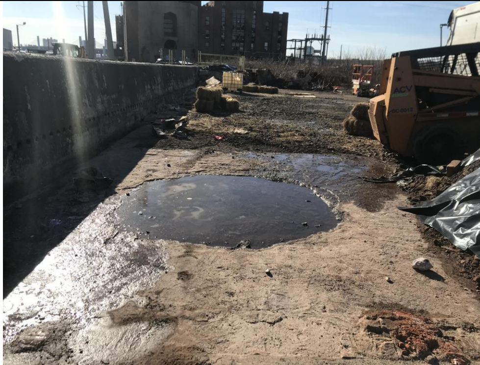
Photo 9: Filled platform area after surface cleaning. Note concrete slab on-grade with circular sand/rubble filled opening in the center. This area will be covered with the 4-foot thick suitable soil fill barrier layer.
