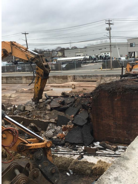
Photo 3: Filled Platform area on right side after removal of the wastewater sump.
