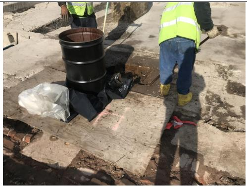
Photo 3: Hand Removal and Drumming of Sump Contents to 1 Foot Deep – 01-15-2020
