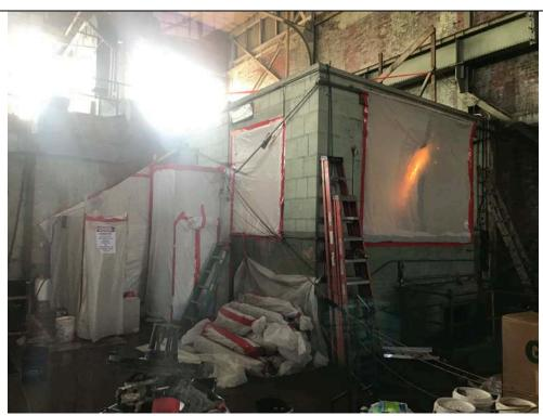
Photo 4: 5/31/2019, Station B interior asbestos abatement containment.
