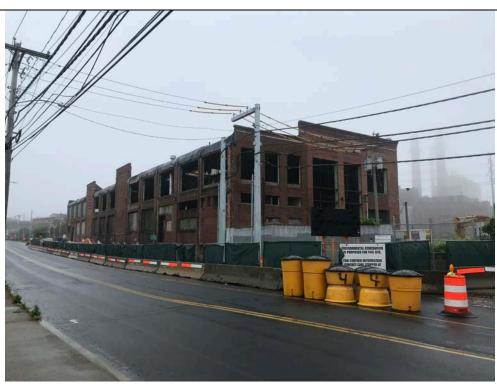
Photo 10: 6/20/2020, Exterior windows removed from the western and part of the northern side of Station B.
