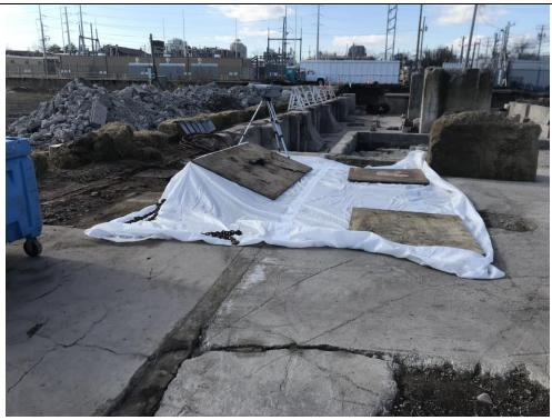
Photo 9: Sump Covered with Poly-Sheeting and Plywood 02-03-2020
