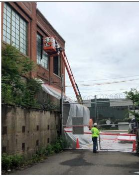
Photo 11: 6/21/2019, Asbestos abatement contractor removing exterior windows from the eastern side of Station B.
