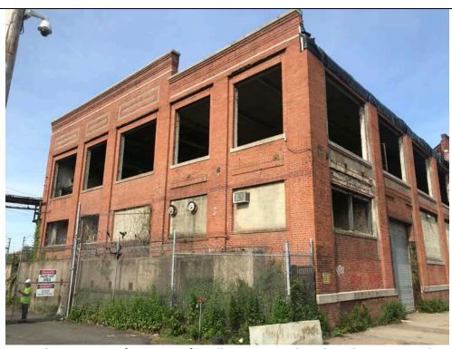
Photo 12: 6/28/2019, Northeast corner of Station B after all exterior windows have been removed.
