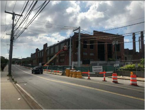
Photo 9: 6/14/2019, Asbestos abatement contractor removing exterior windows from the northern side of Station B.
