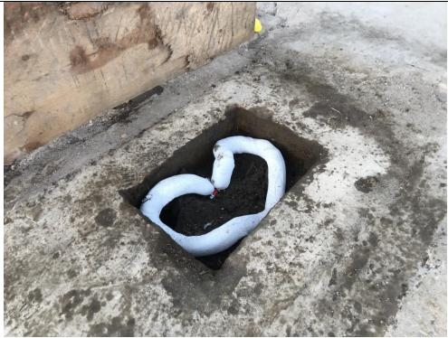
Photo 5: Absorbent Sock Placed inside Sump – 01-16-2020
