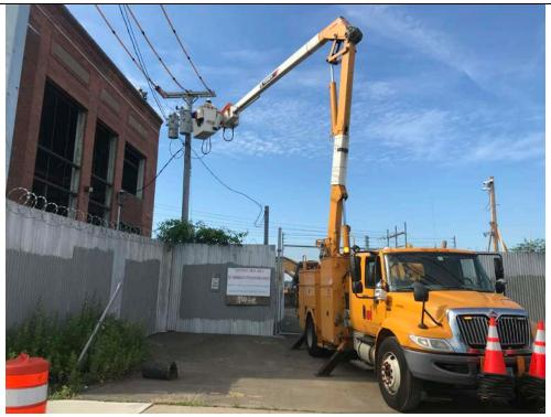
Photo 13: 7/3/2019, United Illuminating disconnecting 480-volt electrical service to English Station.
