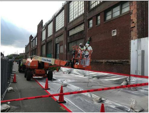
Photo 7: 6/14/2019, Asbestos abatement contractor preparing a work area on the northern side of Station B.
