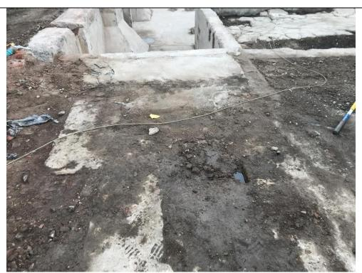
Photo 2: Initial Hand Excavation and Discovery of Free Phase Oil. Oil Sample (TRC-AOC-1-OIL-01) Collected – 01-14-2020
