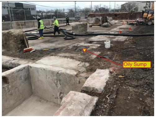
Photo 1: Sump Location Looking East along South Wall of Station B – 01-14-2020
