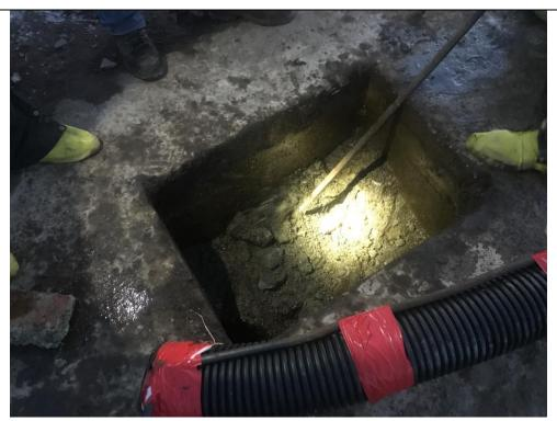
Photo 6: Loosening Sump Contents during Turbo-vac Removal – 01-22-2020
