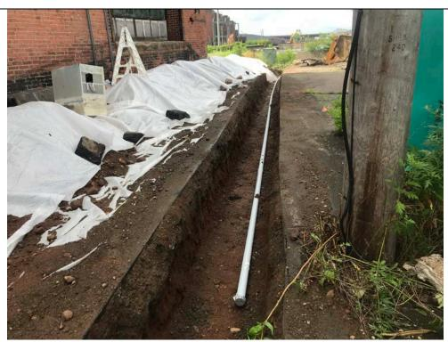
Photo 14: 7/12/2019, Conduit trench for the realignment of 480-volt service.
