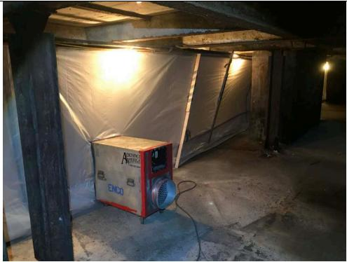
Photo 3: 5/17/2019, Station B basement asbestos containment and negative air machine with HEPA filter.
