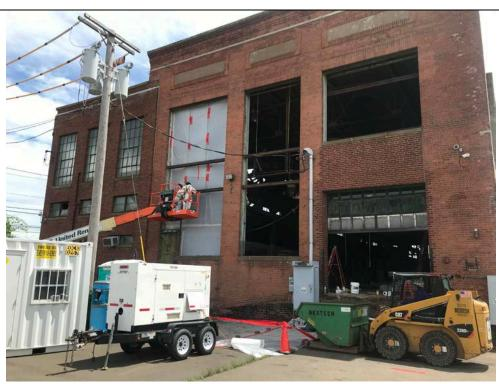
Photo 6: 6/11/2019, Asbestos abatement contractor removing exterior windows from the western side of Station B.
