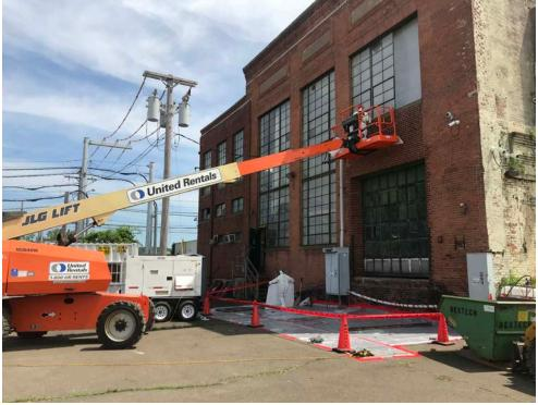
Photo 5: 6/7/2019, Asbestos abatement contractor removing exterior windows from the western side of Station B.
