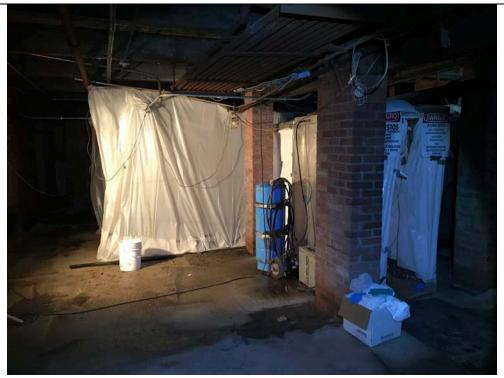
Photo 1: 5/15/19, Station B basement asbestos abatement containment.
