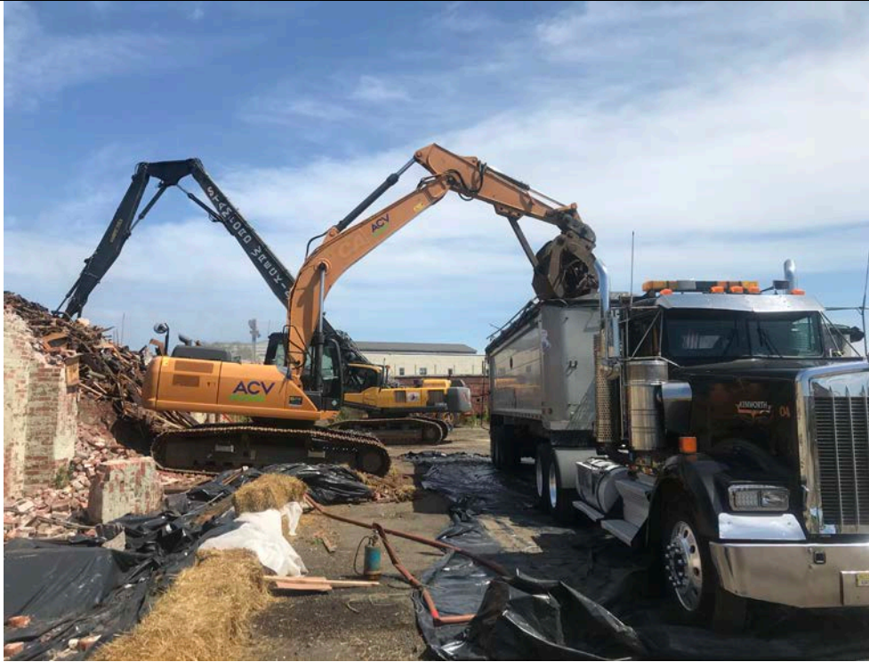
Photo 29: 8/20/2019, Station B demolition debris waste load out.
