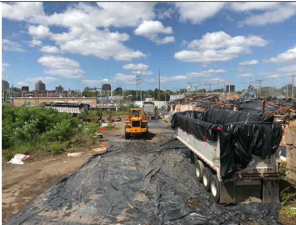
Photo 32: 8/26/2019, Station B demolition debris waste load out.
