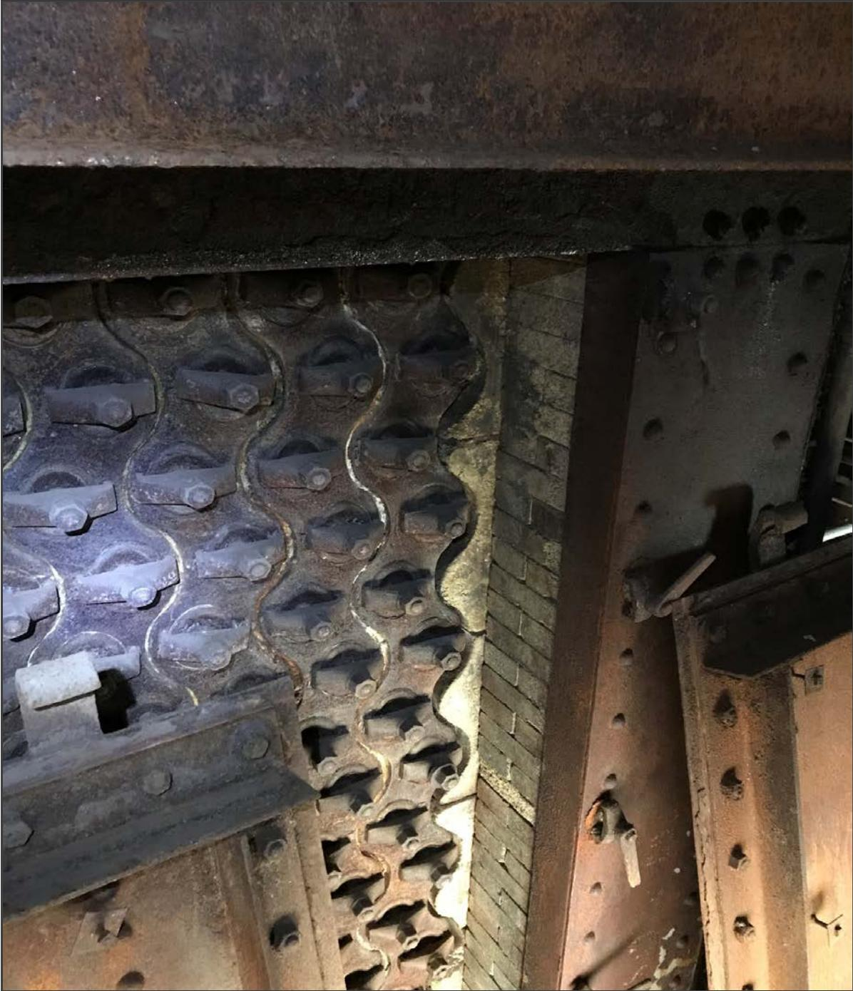
**PHOTO 1 – 2<sup>nd</sup> Floor Boiler 1-12 Area – View of Boiler Ribs**
