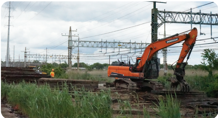
UI crews replace critical infrastructure in the Milvon to West River phase of grid reconstruction. Similar work is slated for the Fairfield to Congress phase, currently in design.
