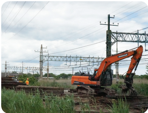
UI crews replace critical infrastructure in the Milvon to West River phase of grid reconstruction. Similar work is slated for the Fairfield to Congress phase, currently in design.
